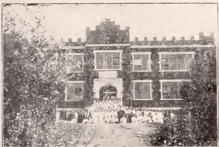
The new Seminary Building.
